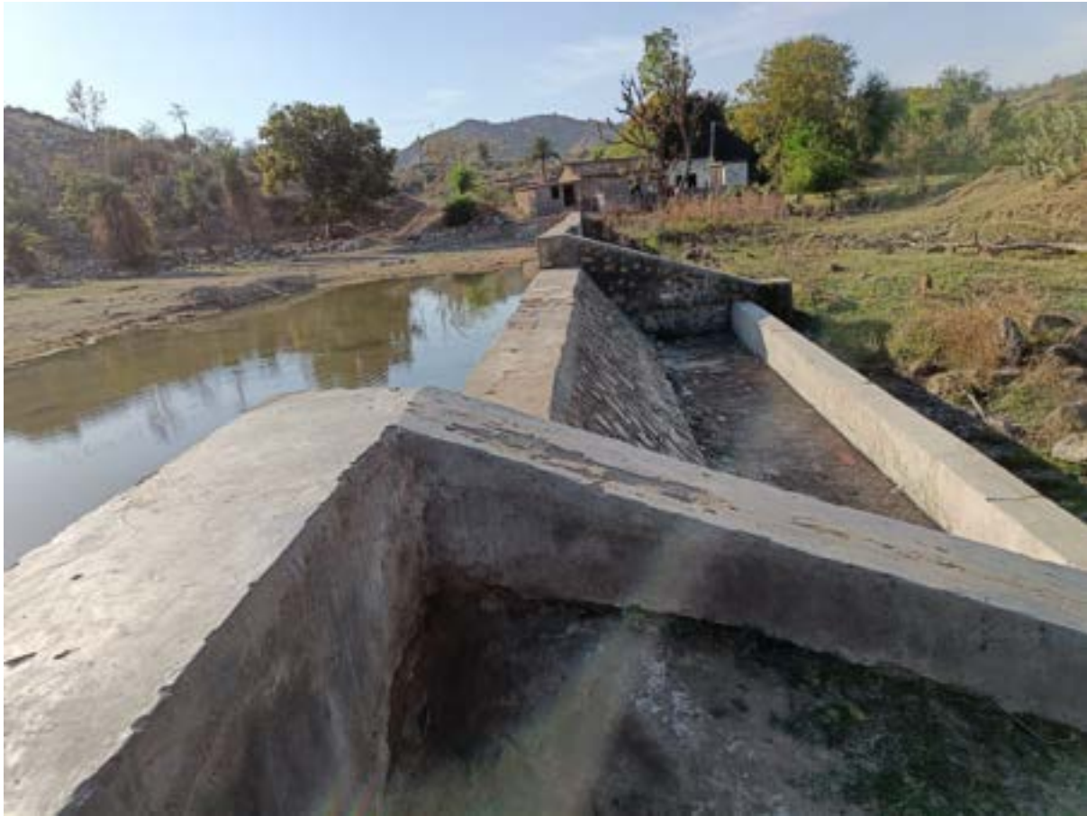
Plate 1. Check dam strengthened in Mandli watershed, Udaipur district, Rajasthan
