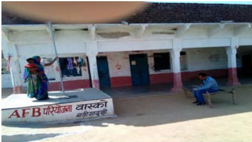
Roof rainwater storage tank constructed with the support of AFB project.
