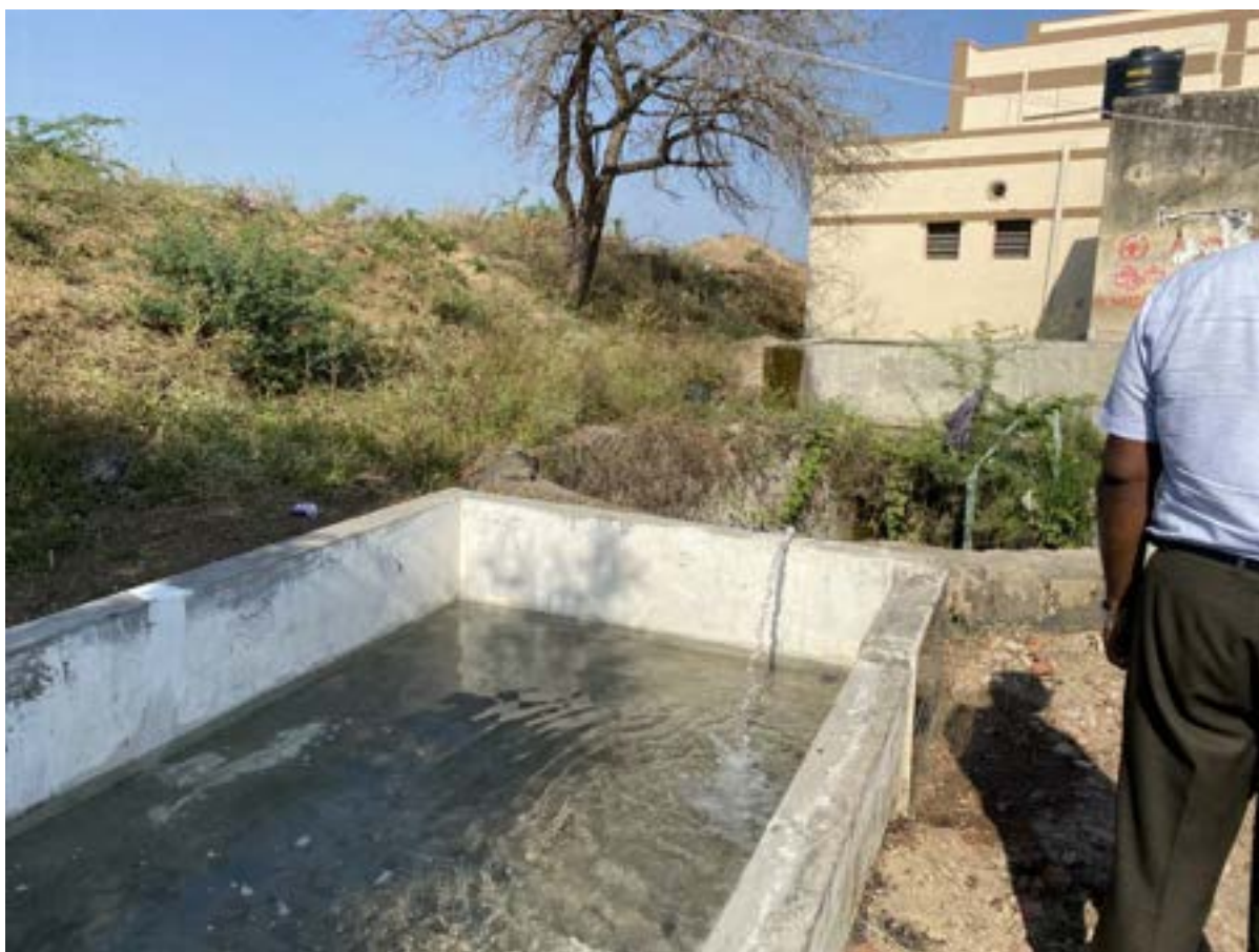
Plate 2. Water tank with drinking water facility for animals at Chithalai watershed, Madurai district
