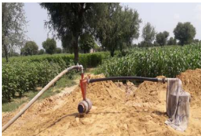
Photo 8.6: A typical set up of tube well with fertilizer mixer and main pipeline
