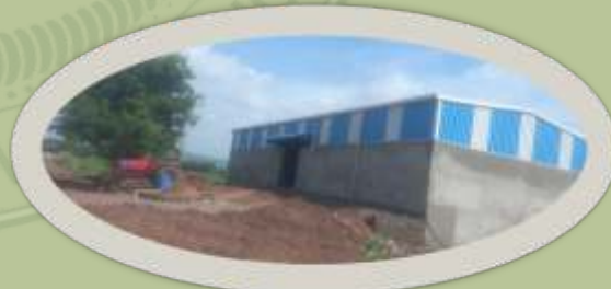
500 MT Warehouse constructed under TRICOR Assistance by TRN FPCL
