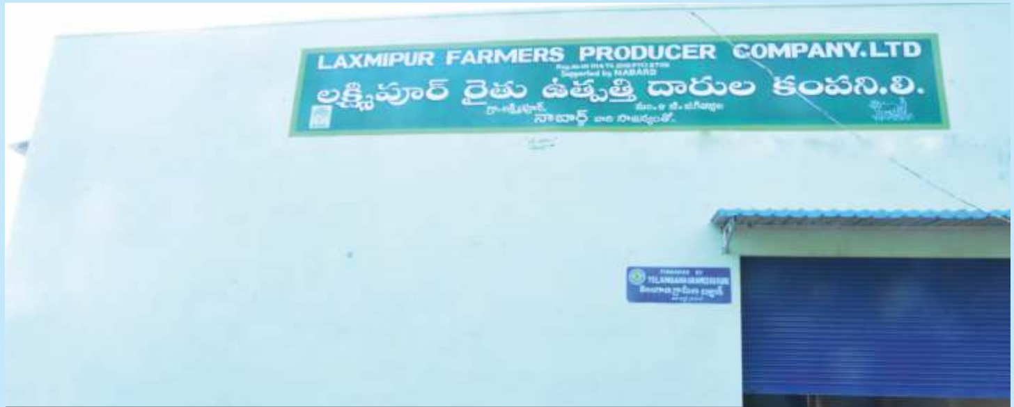
750 MT Warehouse constructed with credit assistance from TGB
