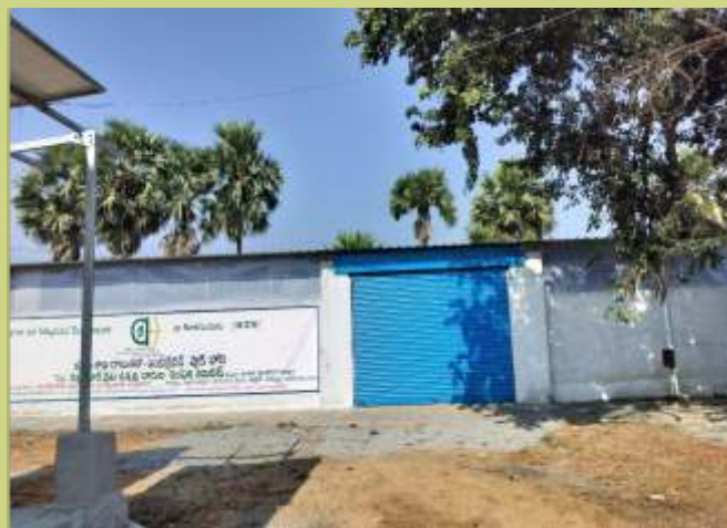
Construction of Integrated Packing House under Mission for Integrated Development of Horticulture at Kattangur FPCL, Nalgonda
