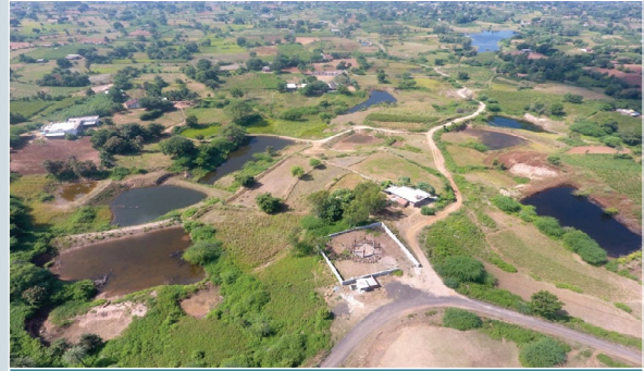
Drone image of Bijalpur Haliya village showing various percolation tanks
